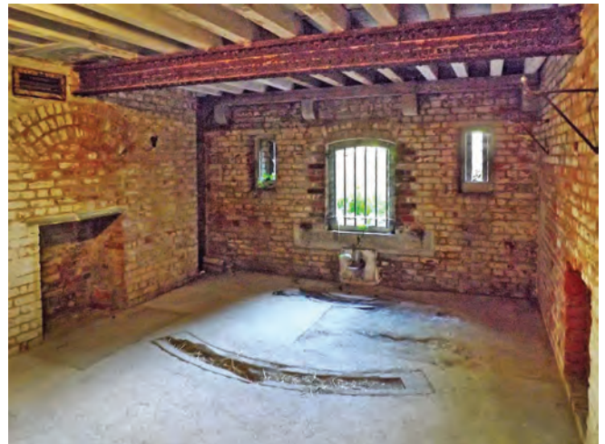
A gun position in a caponier at Fort Widley. Note the mounts in the floor to manoeuvre the gun
